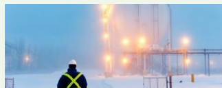
Electrolyzer in Quebec
